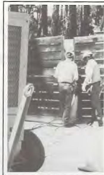
Temporary power is linked up by Presidio of Monterey engineers. A fence was put around the generator to help baffle the noise.
