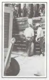
Temporary power is linked up by Presidio of Monterey engineers. A fence was put around the generator to help baffle the noise.
